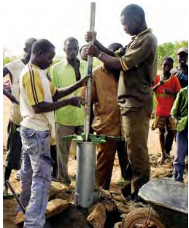
Installation and assembly of a pump.
